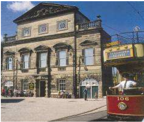
Facade of the old Derby Assembly Rooms at Townend Picture from the Crich Tramway Guide Book
